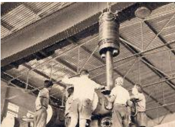
Figure 12 Lowering the piston down the liner
