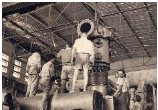
Figure 9 Lowering of cylinder casing and liner into the frame
