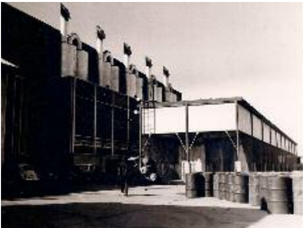
Figure 4 Doha Power Station showing fin fan coolers on the right
