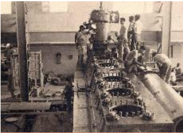
Figure 10 Alternative view of the fitting of a cylinder casing
