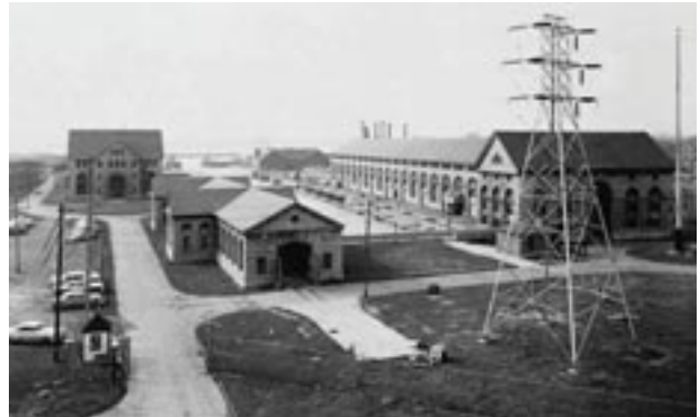
Figure 2 The Adams Power Plant before most of it was demolished. The transformer house is seen centre-left.
