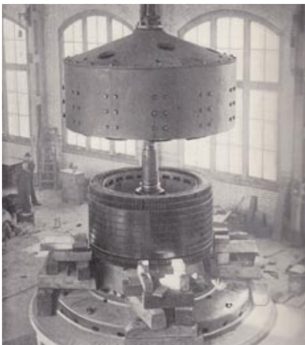
Figure 6 A field ring ready to be lowered onto a generator shaft
