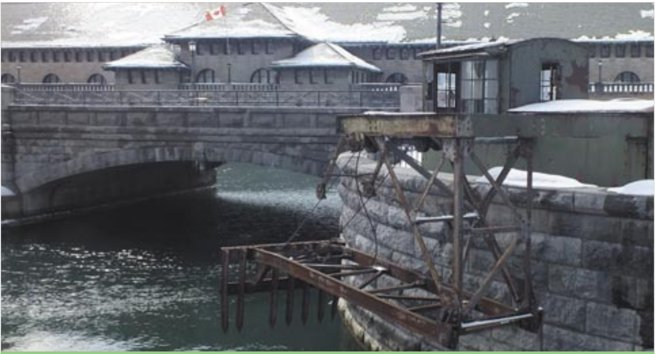
Figure 15 Entrance to the forebay from the Upper Niagara river
