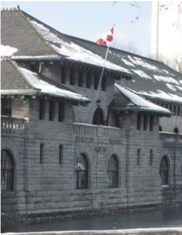
Figure 22 The name of Canadian Niagara Power together with the flag is prominent on the front face of the power house
