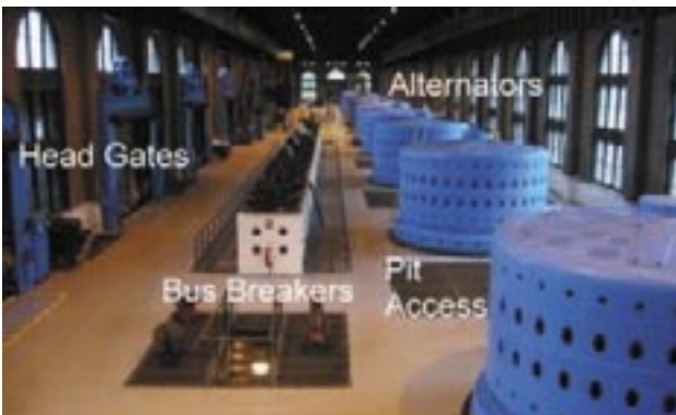
Figure 17 Interior of the powerhouse
