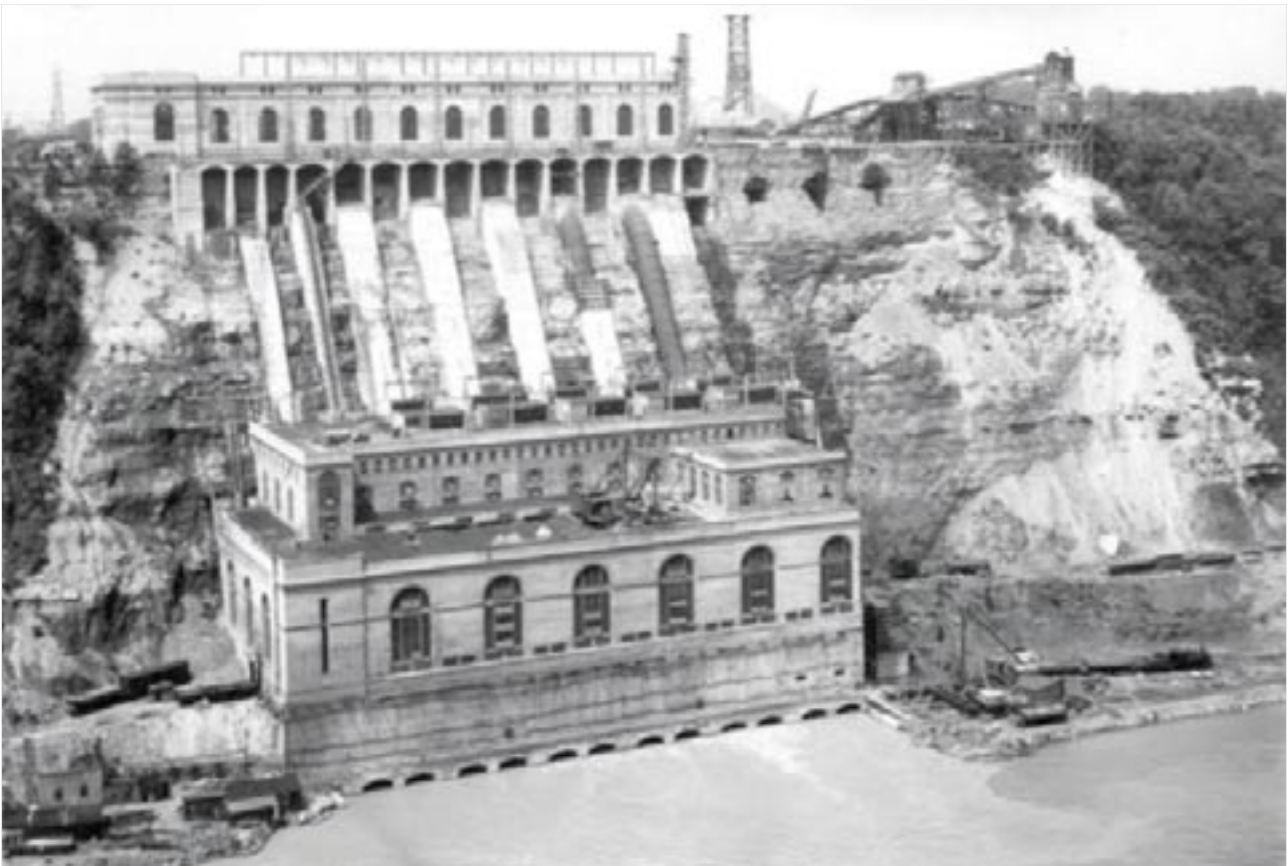
Figure 10 Construction at the Sir Adam Beck Power Generating Station - June 1923
