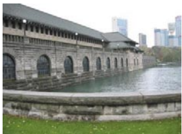
Figure 12 Rankine powerhouse with forebay, (current photo with high rise behind)
