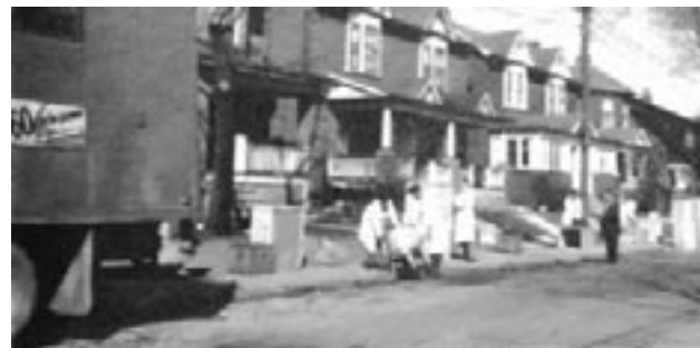
Figure 8 During the 1950s all of Ontario was systematically converted from 25Hz power to 60Hz power. Trucks like those shown here came through each neighbourhood converting motors to the new frequency. You'll note here the sign on the truck "60 cycle power for progress".
