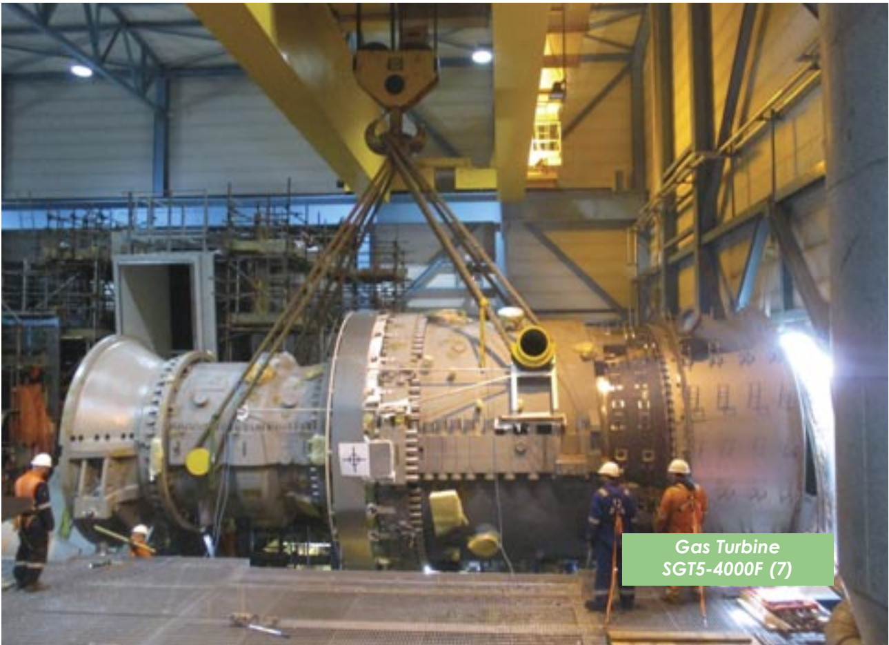
Figure 5: New GT being installed on concrete foundation pads
