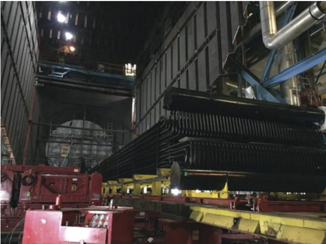
Figure 8: New HRSG modules ready for lifting into place
