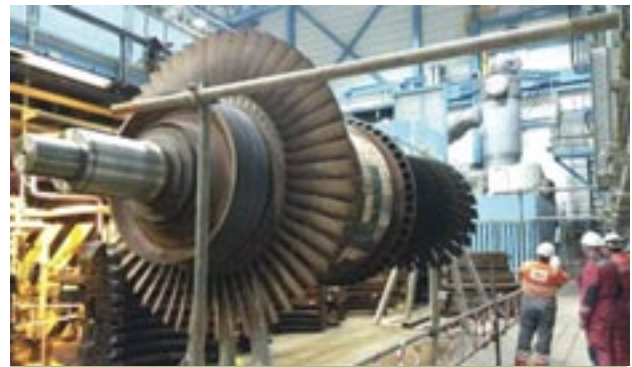
Figure 2: Removal of Siemens V94.3A gas turbine
