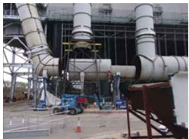
Figure 10: ACC steam duct pipework modification
