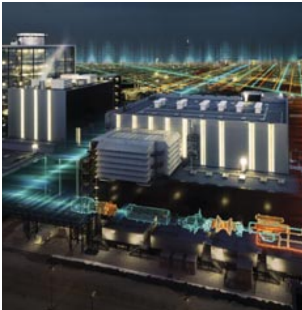
Copyright © Siemens Energy, 2019
