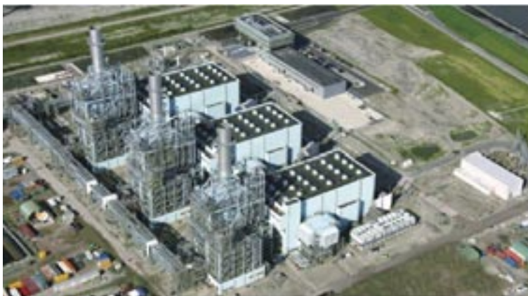
Figure 13 Vattenfall's Magnum power plant in Groningen, the Netherlands
