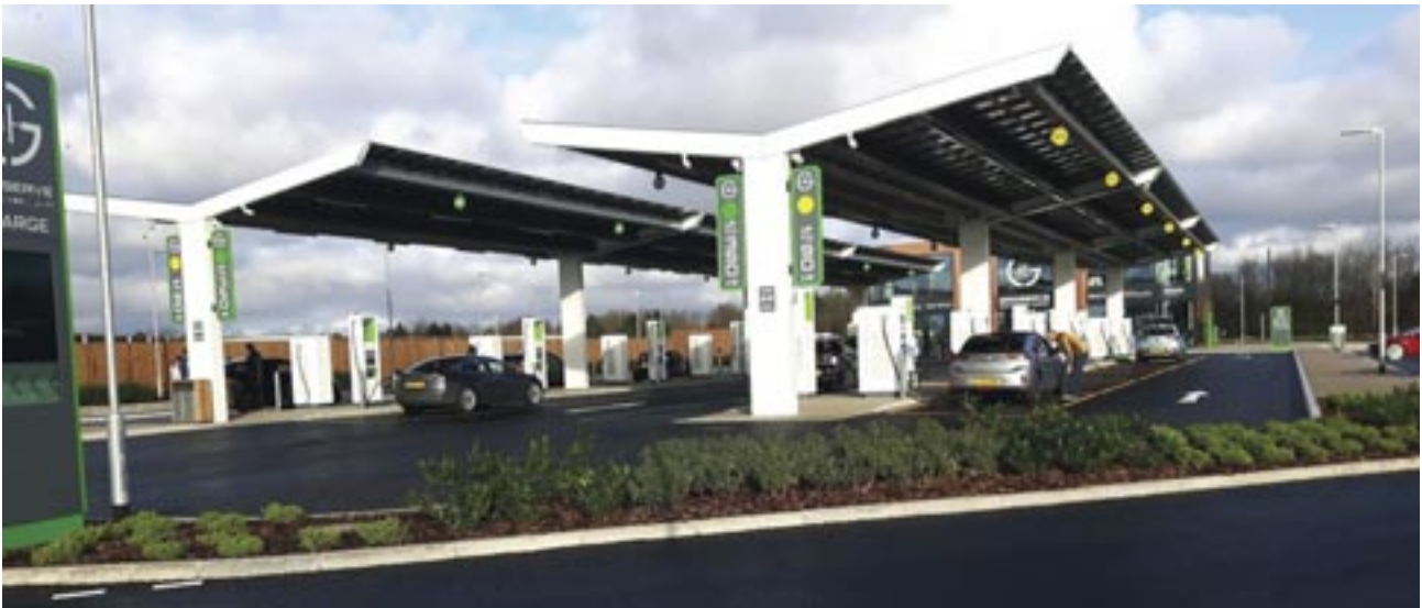
Figure 6: Gridserve Chelmsford site
