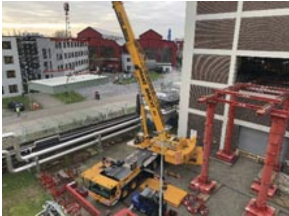
10:00 h: and brought into the building
