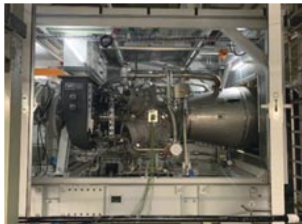
The gas turbine is installed
