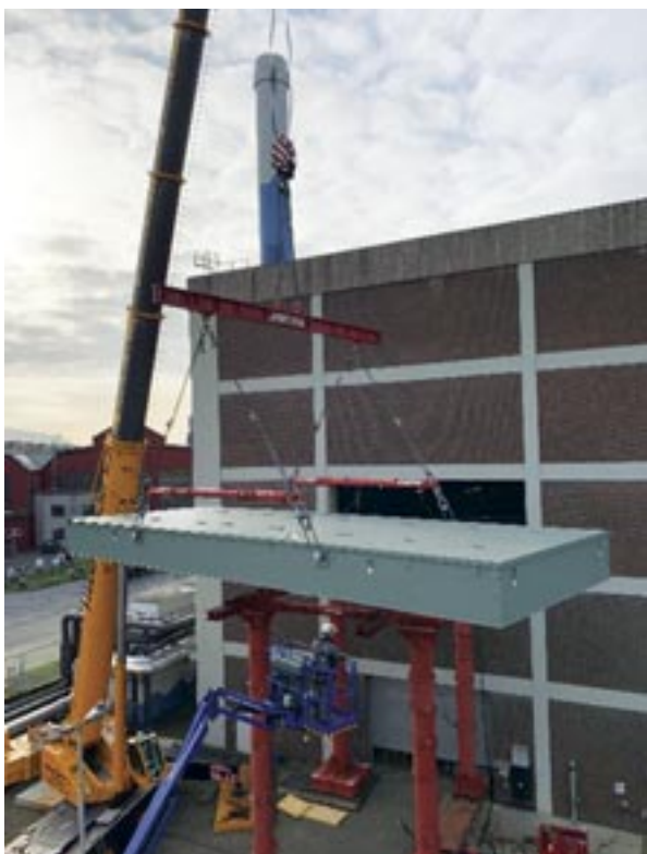
11:00 h: 2nd base frame is lifted
