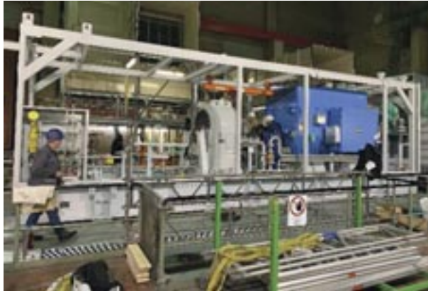
The enclosure being erected
