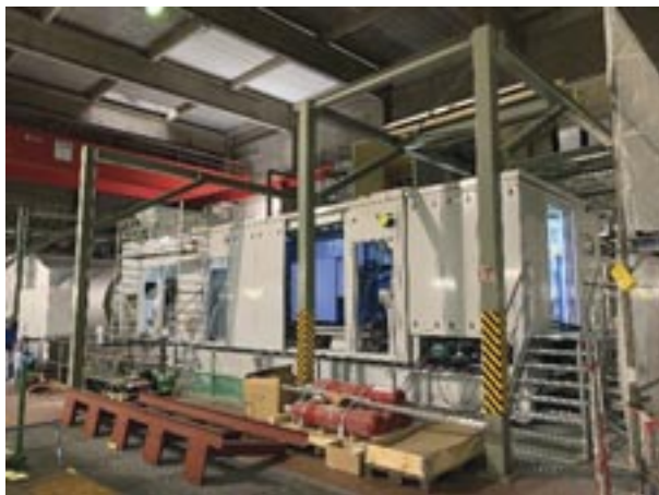
The insulation is applied & cabling conducted
