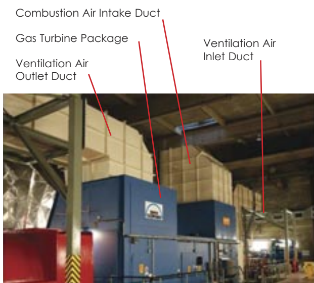
Figure 1: The FT8-Package in power plant HKW II of evo (left) and general layout of the train (right, after [6])
