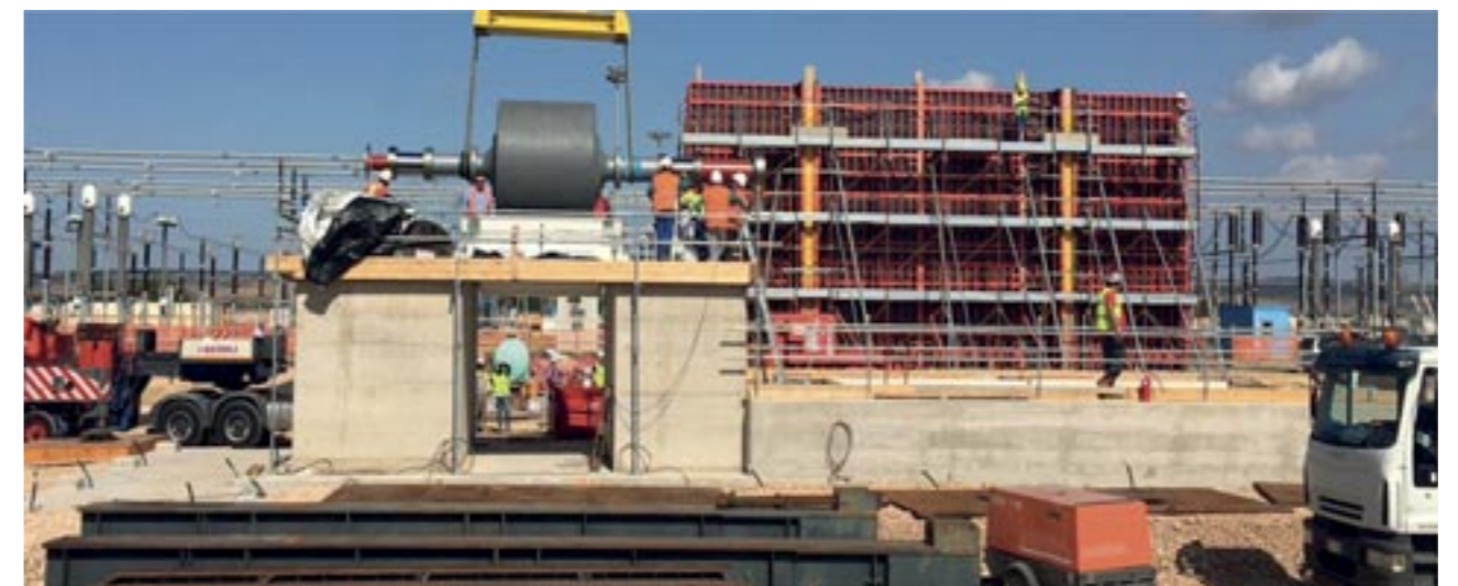
Figure 10 – Site photos - Flywheel site assembly
